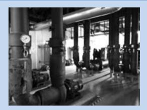
In 2017, Taizhou FDZJ reconstructed the water chillers and made two of them operate in network, by which electricity could be saved 758,552KWh on average per year. Besides, Taizhou FDZJ adopted temperature control, and the control temperature of HVAC system was set to be 23±2°C in summer and 21±2°C in winter, which could further increases energy efficiency.
