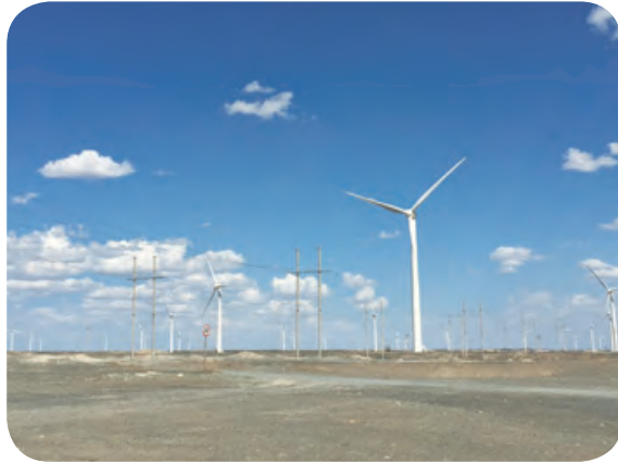
Liuyuan Wind Project
