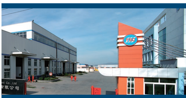
Offshore Qingdao Facility in China
