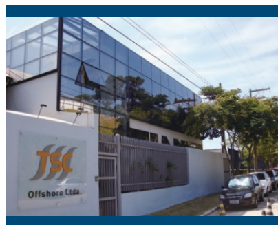
Macaé Facility in Brazil
