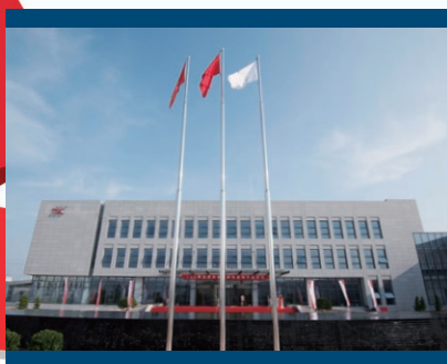
Qingdao Manufacturing Facility in China
