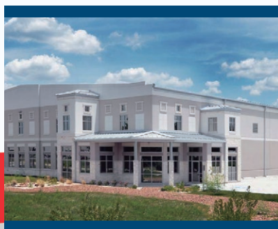
Houston NHR Facility in USA
