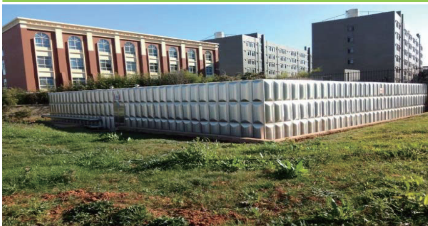
Yunnan School's Water Storage Pool with Storage Capacity of 1,000 m 3
