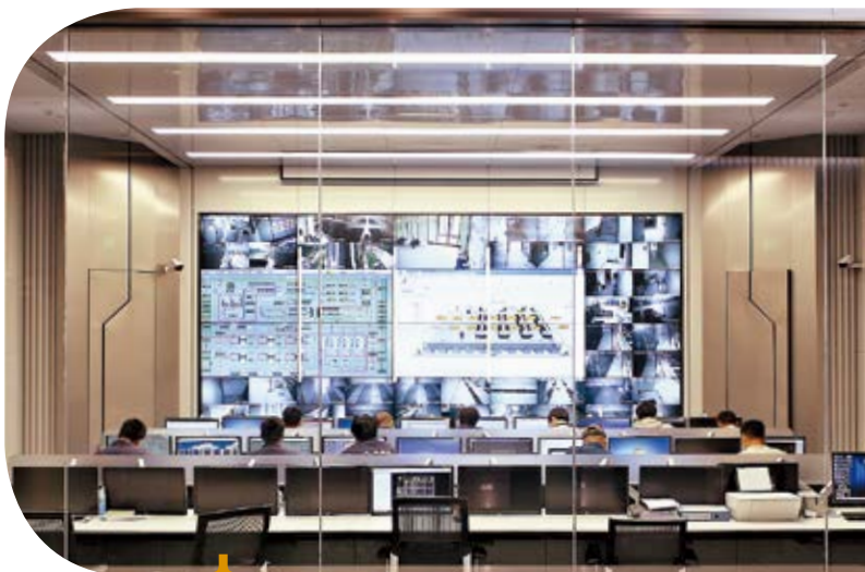
TGT Beijing Data Centre 1 started operating in 2017.
