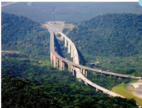
Deployed a turnkey wireless solution for the longest and busiest highway tunnel system in Brazil
