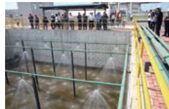
The 100,000-cubic-metre accident buffer pool and its supporting collection system
