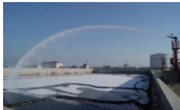
The 100,000-cubic-metre accident buffer pool and its supporting collection system
