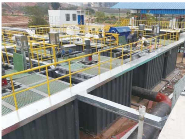
Everbright Nanning Shuitangjiang Project
