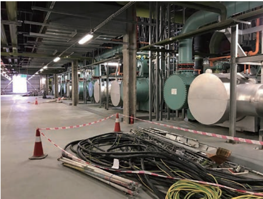
Provision of operation and maintenance services for energy centres of hotel complex
