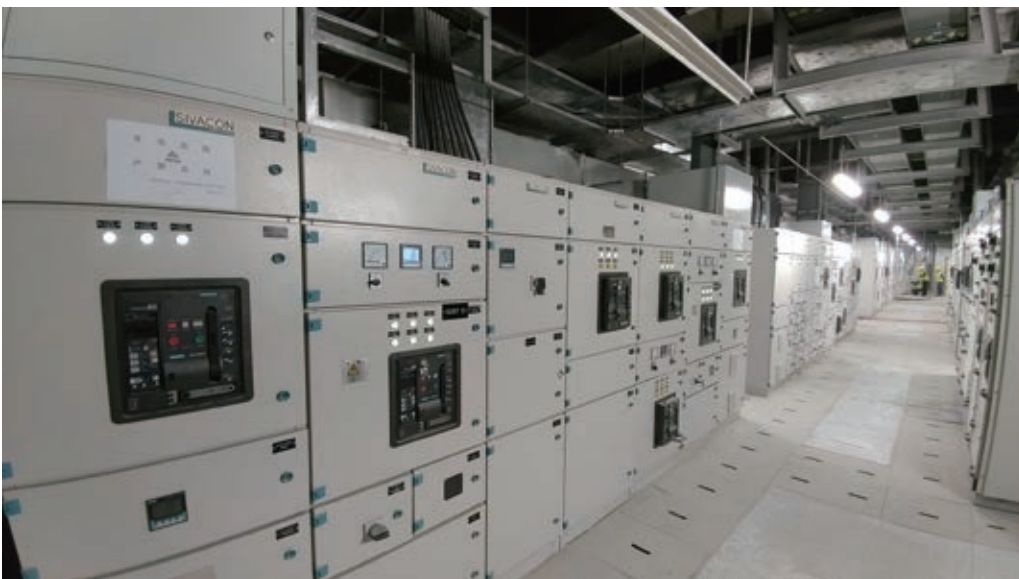
Power distribution system services and works for the Hong Kong-Zhuhai-Macau Link Bridge – Macau Port of Entry (Customs and Immigration)
