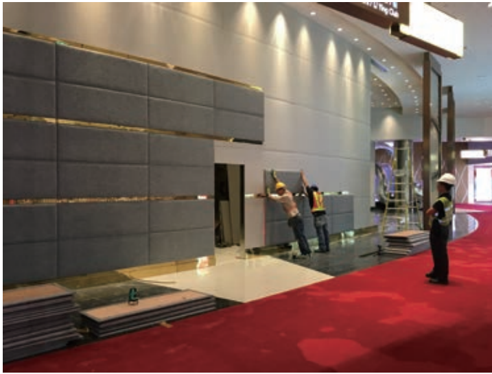
Renovation works in major casinos
