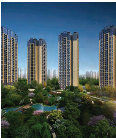
Chongqing Danzishi Project, Phase 2
