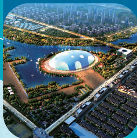
Tianjin • Tian Shan Waterpark
