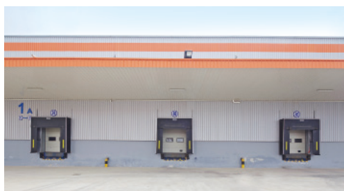
Avant-garde loading facilities
