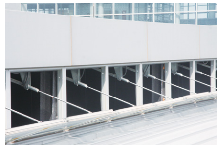
Electrically-opened windows in National Convention Centre
