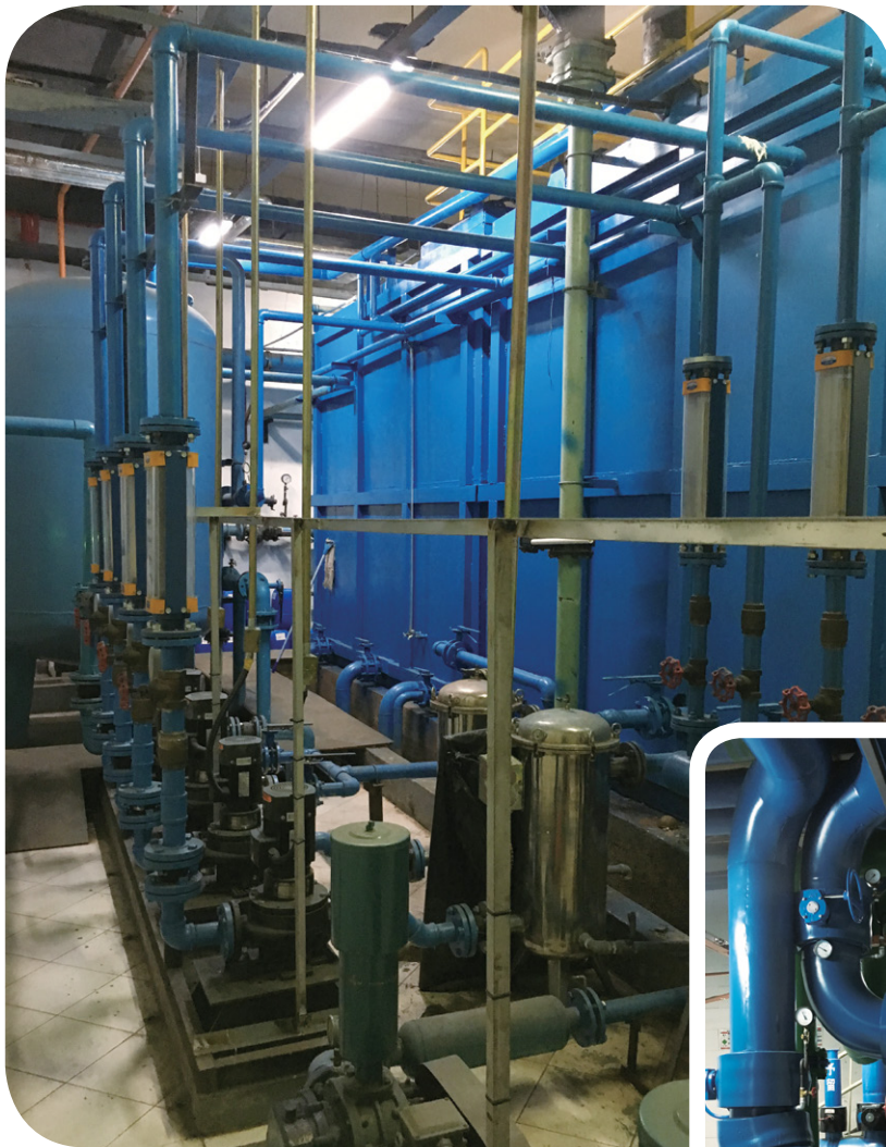
Overview of cooling water recycle equipment
