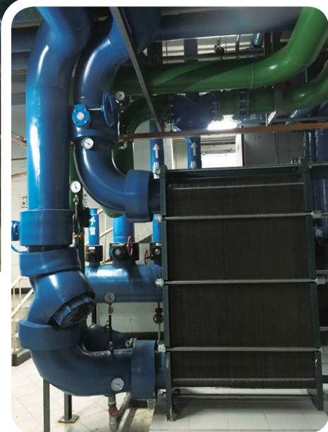
Cooling water recycle equipment
