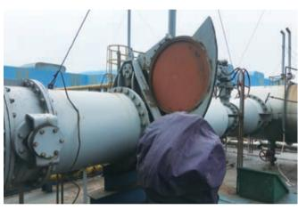
All gas pipelines with a diameter of less than 1.8 meters were upgraded to be equipped with electric blind flange valves
