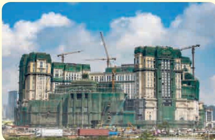
Construction in progress (photo taken in April 2018)
