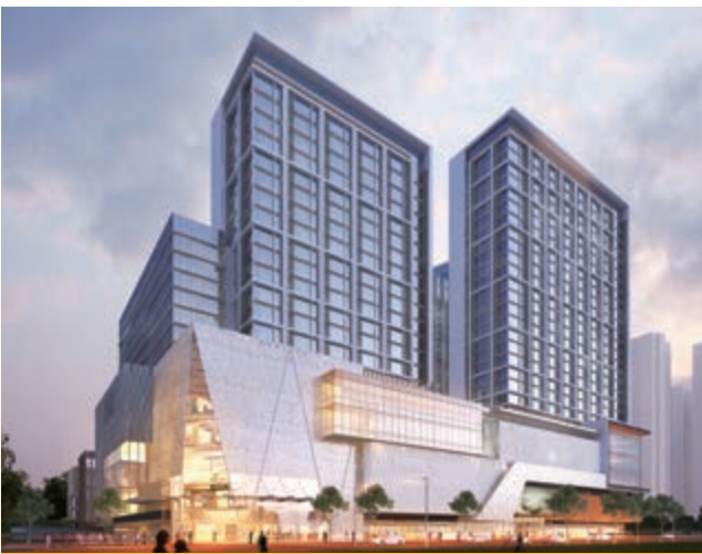
Commercial/office towers of Regal Cosmopolitan City (*)
