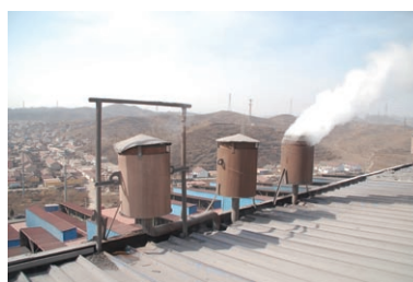
Blow-off silencer for converter drum of Jinxi Special Steel 津西特鋼轉爐汽包放散消間器
