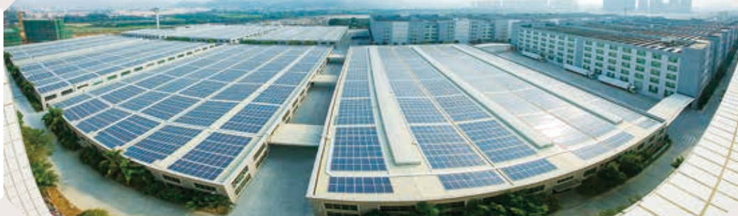
The Rooftop Solar Photovoltaic System
