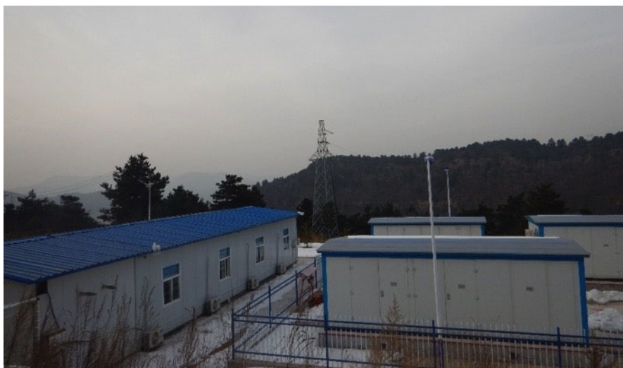
The Power Grid Was Successfully Established and Put into Operation 電網正式建成並投入使用
