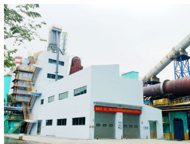
海南昌江年处置三万吨危废协同处置项目 (2018 年 2 月建成) The hazardous waste co-processing project in Changjiang, Hainan with an annual processing capacity of 30,000 tons (construction completed in February 2018)
