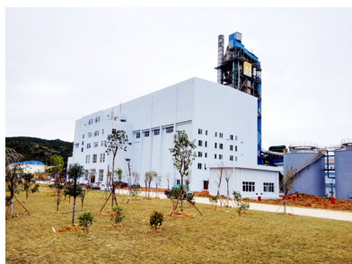
广西田阳县日处置 500 吨生活垃圾协同处置项目 (预计 2018 年上半年建成) The municipal waste co-processing project in Tianyang County, Guangxi with a daily processing capacity of 500 tons (expected completion of construction in the first half of 2018)
