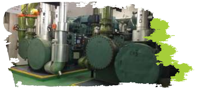
Variable Speed Drive Chillers
