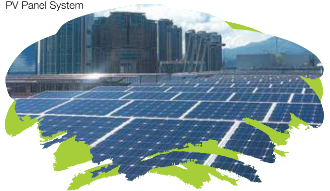
PV Panel System
