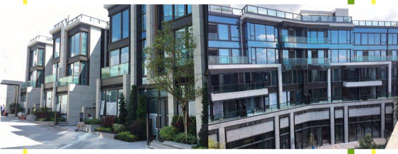
Aluminium window, curtain wall, louver, metal cladding and glass balustrade for St. Moritz at 88 Lai Ping Road, Kau To Shan 九肚山麗坪路88號雲端之鋁窗、幕牆、百葉、金屬飾板及玻璃欄河
