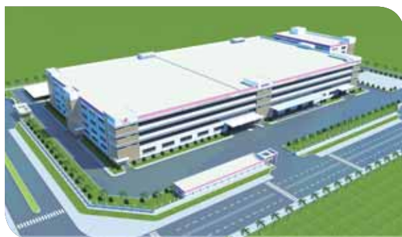
Fifth Vietnamese Facility (Under Construction) 第五家越南廠(興建中)
