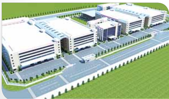
Fourth Vietnamese Facility (Under Construction) 第四家越南廠(興建中)
