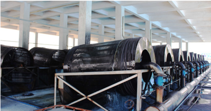
Hydraulic powered rotary screening machines 以水力運行的圓網格柵機
