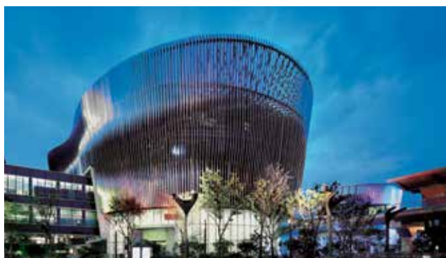
^ Night view of THE HUB
