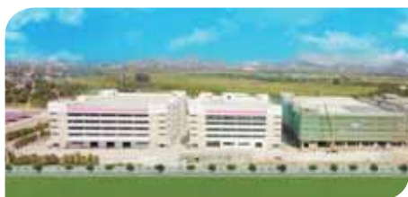
Vietnam Factory D (Under Construction) 越南D廠 (興建中)
