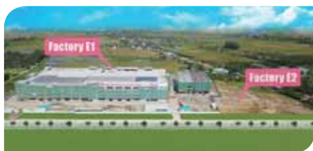
Vietnam Factory E (Under Construction) 越南E廠 (興建中)
