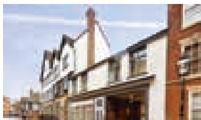
dwell Castle Gate Haus, Nottingham, United Kingdom
