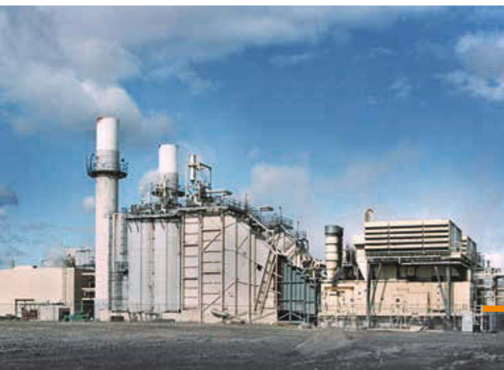
One of the gas-fired power plants owned by Canadian Power in Mississauga, Canada.
