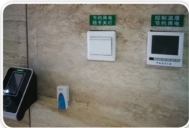
“Saving Electricity” sign posted in PRC subsidiary
