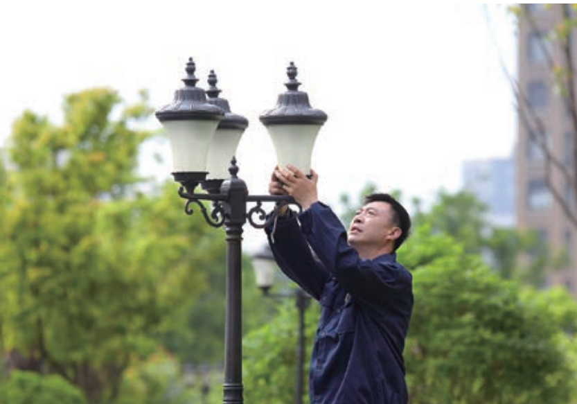
公共設備保養 Public facilities maintenance
