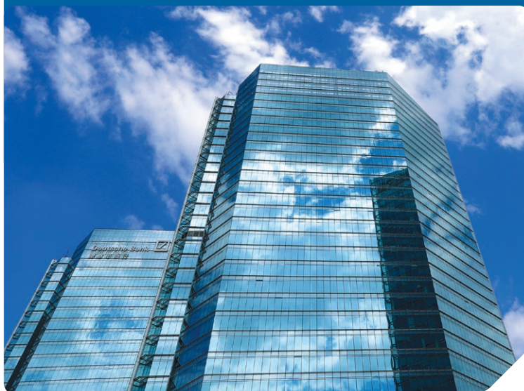
Office Tower 1 & Office Tower 2 China Central Place, Beijing
