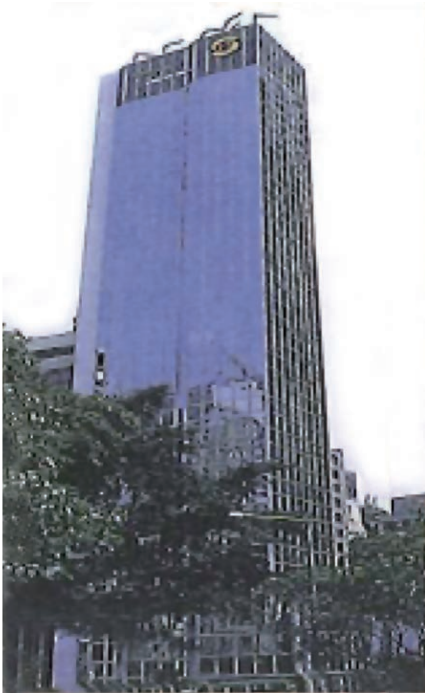
Shun Ho Tower
