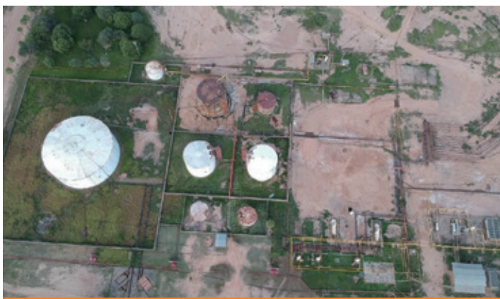
■ Aerial view of Palmar Largo battery tanks
