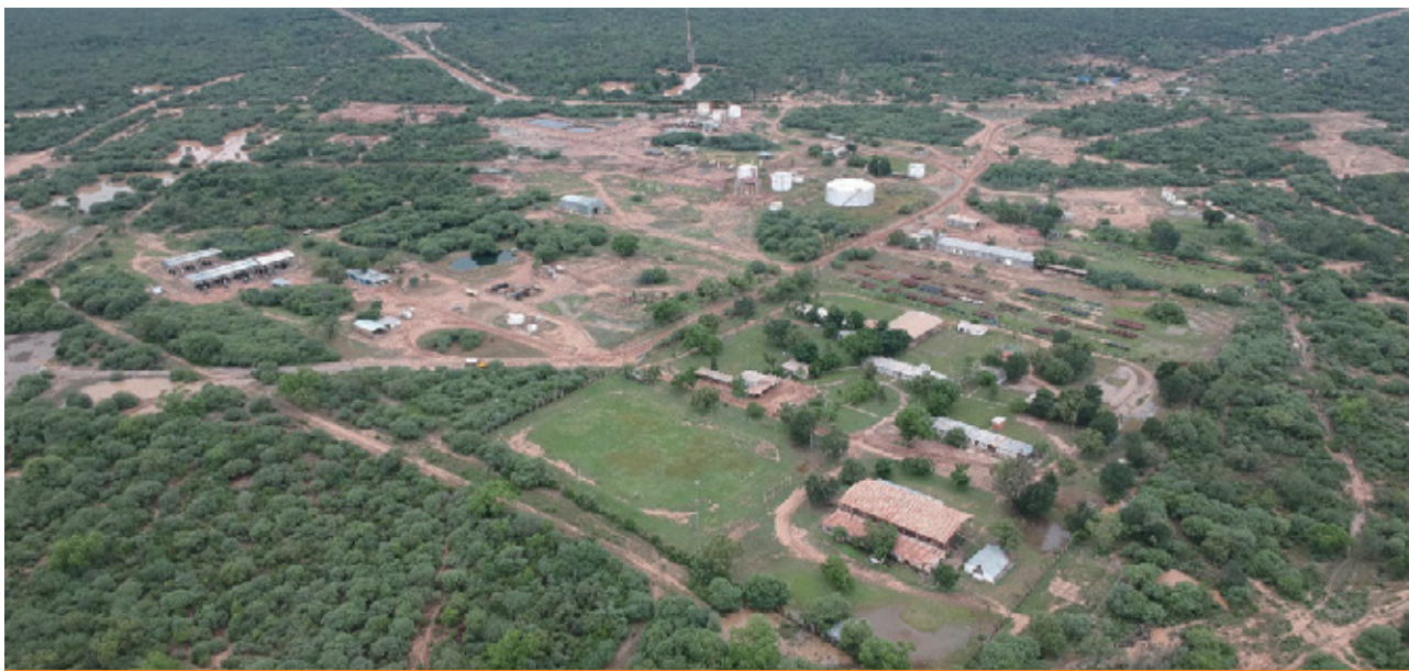
■ An aerial view of the Palmar Largo crude oil production facility
