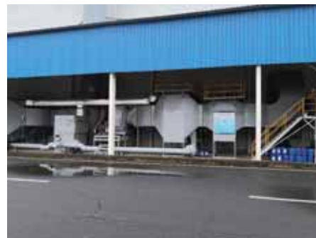
The painting area and emission processing system in one of our factories in Ningbo
