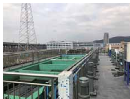
The sewage treatment plant in one of our factories in Ningbo
