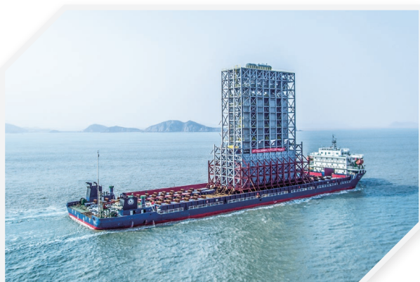
Delivery of unit cracking furnace module for Zhejiang Petrochemical 1,400kta ethylene cracking furnace modules project
