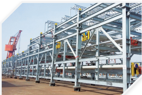
The modularized piperack project in Texas, the United States
