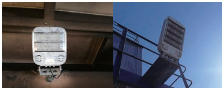
Replacement of lighting equipment for gantry cranes
