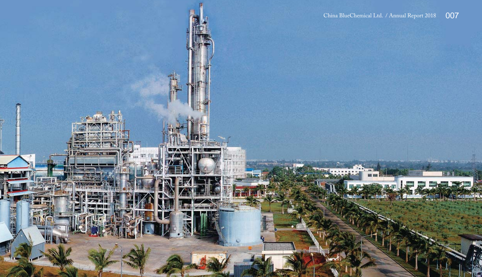
| Hainan Fudao Phase I Plant
