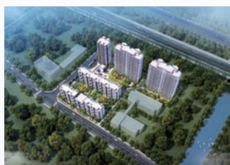
Hangzhou Jiubao Project
