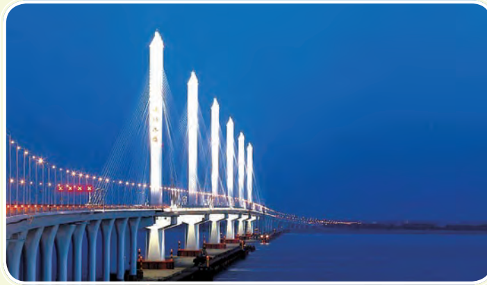
COSCO Kansai Companies Supplying Anti-Corrosion Coatings to the steel structure of Jiaxing-Shaoxing Sea Bridge.
