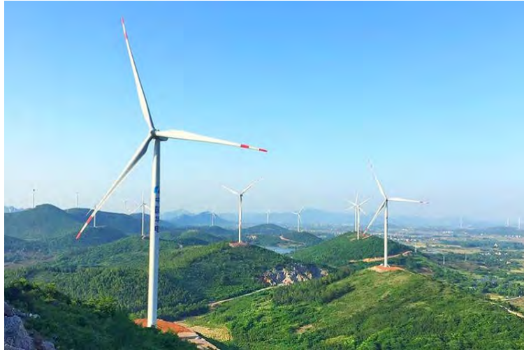
The wind power plants of the Group in Wuwei, Anhui
