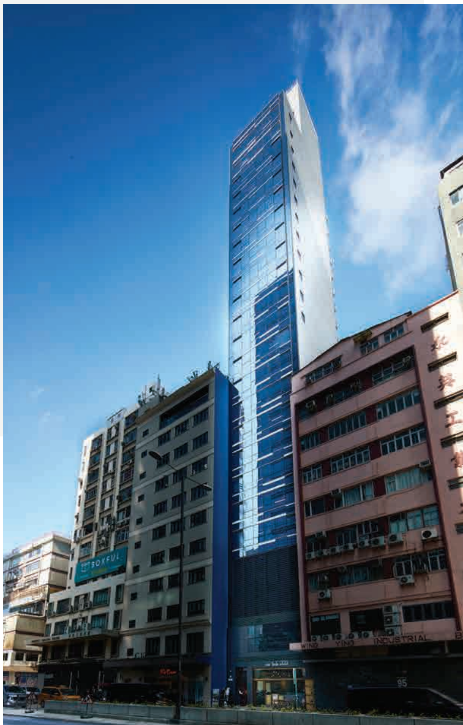
The commercial building was acquired in December 2018
