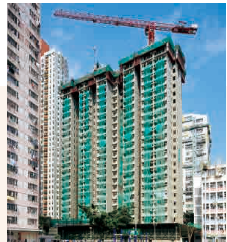
Construction of Public Housing in Chai Wan
