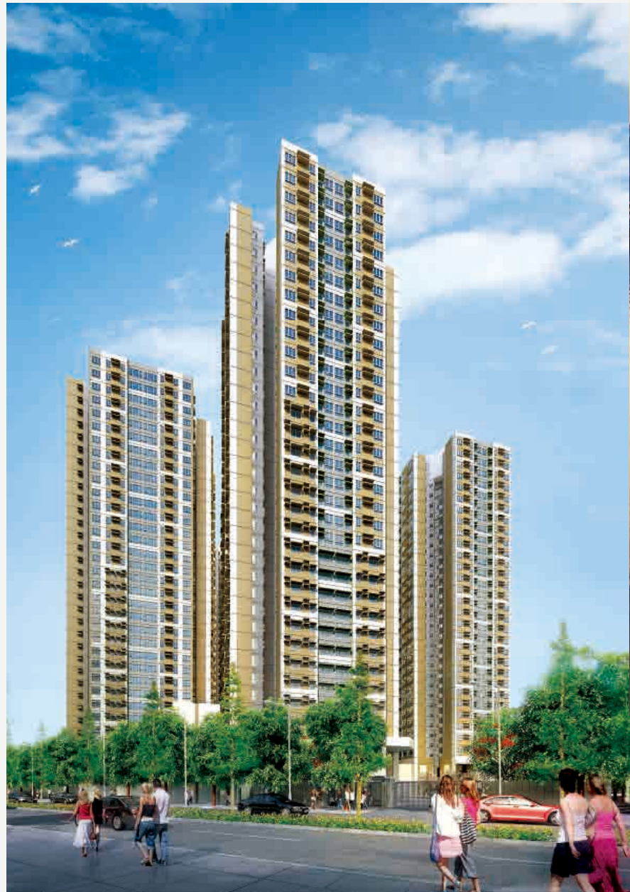
SOC made progress on its major contract in Fan Garden, Fanling
