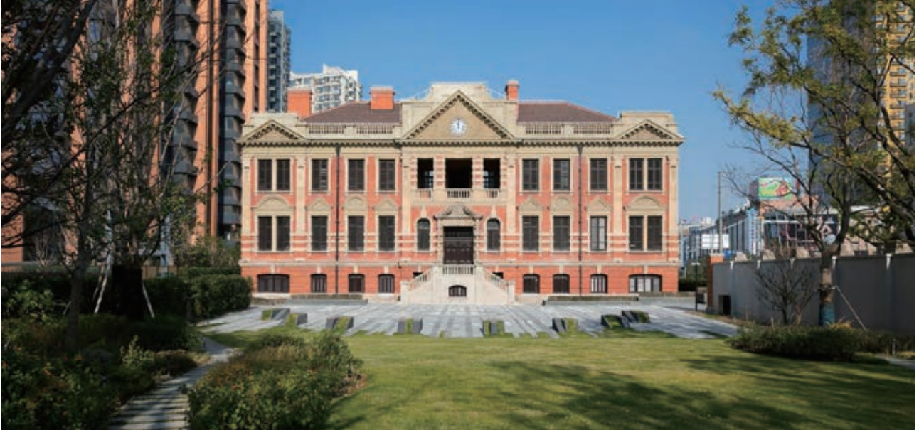
Shanghai General Chamber of Commerce Building
