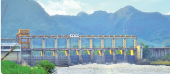
Zuojiang Hydro Project
