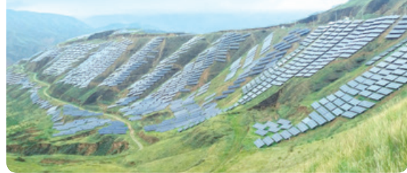
Ledu Solar Project
