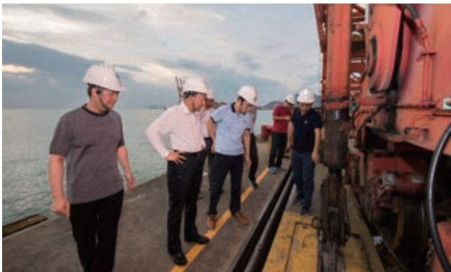
On-site safety inspection by the management
