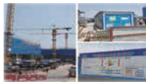
Visiting the Green Building Construction
