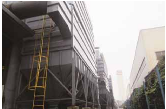
Welding dust control and treatment for the structural component plant in the north area of Zhengzhou Coal Mining Machinery Comprehensive Equipment Co., Ltd. 鄭州煤機綜機設備有限公司北區結構件分廠焊接煙塵治理
