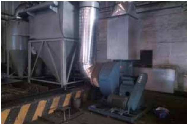
NC-cutting dust treatment for the structural components plant in the north area of Zhengzhou Coal Mining Machinery Comprehensive Equipment Co., Ltd. 鄭州煤機綜機設備有限公司北區結構件分廠數控切割煙塵治理
