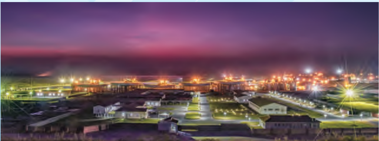
CNMC Luanshya Muliashi Leach Plant at Night
