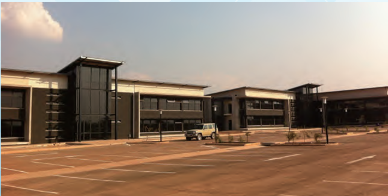
CNMC Huachin Mabende Office area in Lubumbashi in DRC
