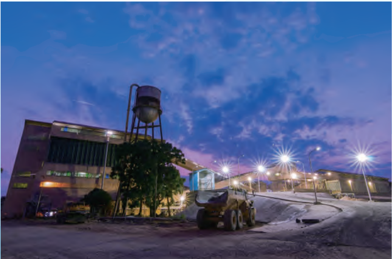
CNMC Luanshya Processing Plant at Dusk
