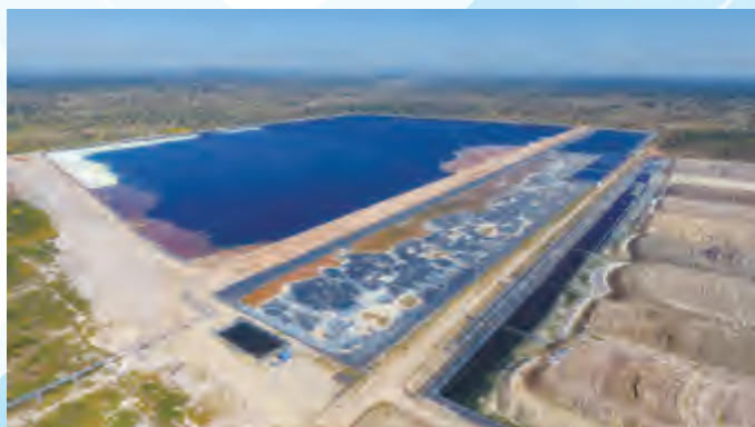
Muliashi tailings dam
