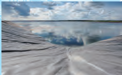
Green tailings pond covered with HDPE film in Luanshya
