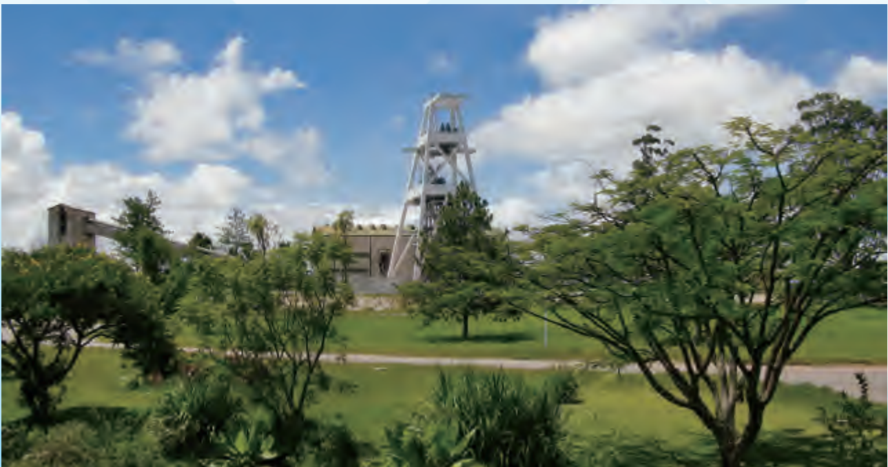
Central auxiliary shaft of Chambishi West Mine
