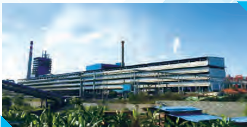
A general view of the exterior of Chambishi Copper Smelter
