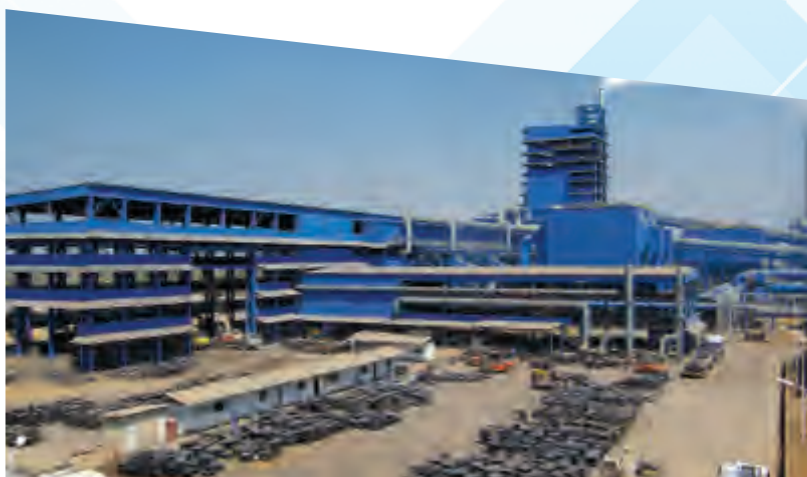
A general view of the interior of Chambishi Copper Smelter
