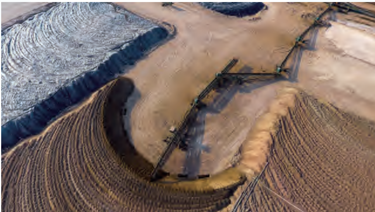
A bird view of the self-propelled heap leaching technology at CNMC Luanshya
