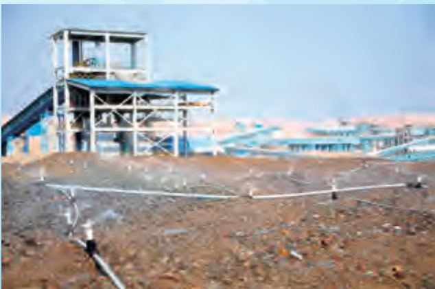
Spray leaching operations in the No.1 stockpile of heap leaching system of Muliashi Project
