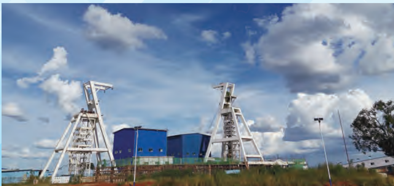
Main and service shaft of Chambishi Southeast Mine
