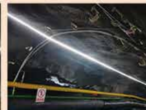
Lighting belts and automatic spray device
