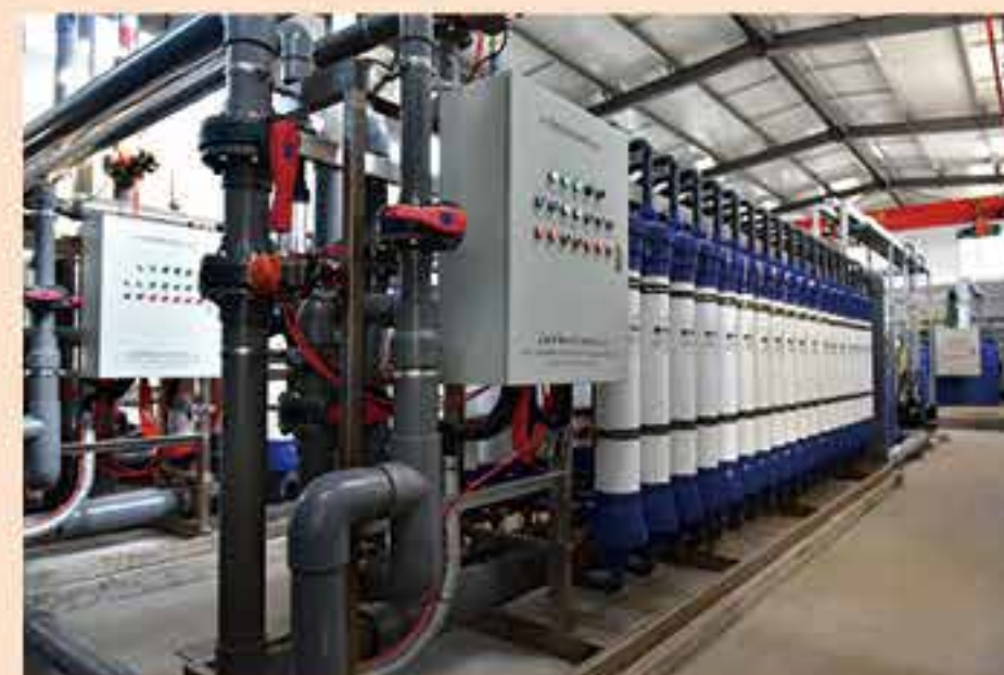
Jiaojia Gold Mine "Downhole Water Products Water Treatment System", the first gold mine underground ultrafiltration + reverse osmosis double membrane step treatment and its automatic control technology and equipment
