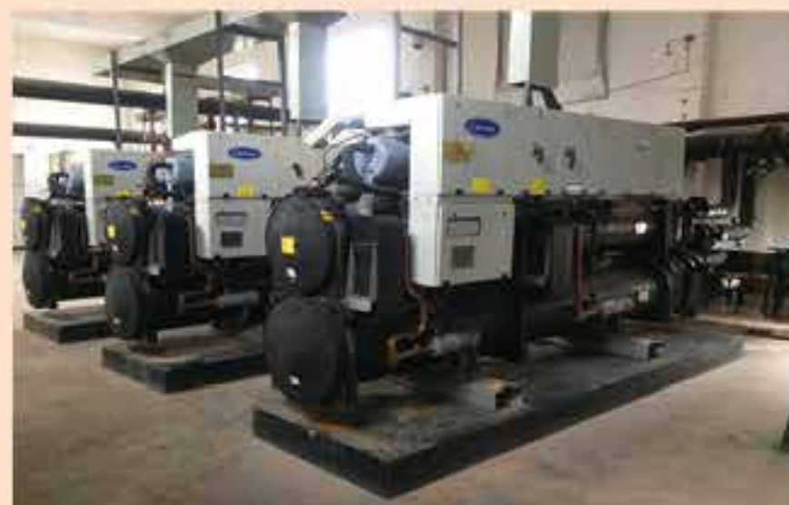
Water source heat pump equipment of Guilaizhuang Mining Company
