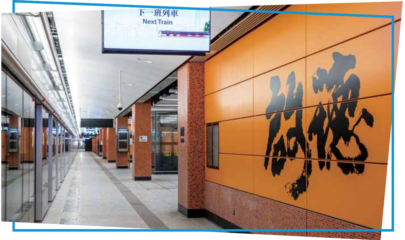
MTR Contract No.1108 — Shatin to Central Link: Kai Tak Station and Associated Tunnels 港鐵合約編號1108 — 沙中綫：啟德站及相關隧道工程
