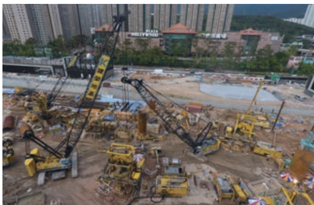
Foundation piling works at Diamond Hill
