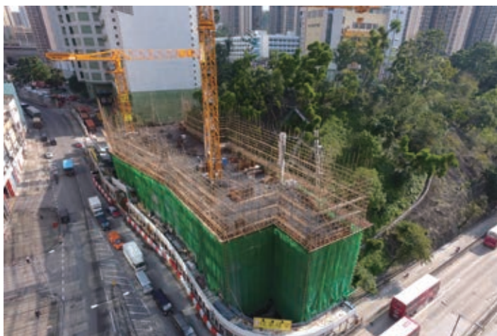
K.C.T.L. No.495, Kin Chuen Street, Kwai Chung – construction works in progress
